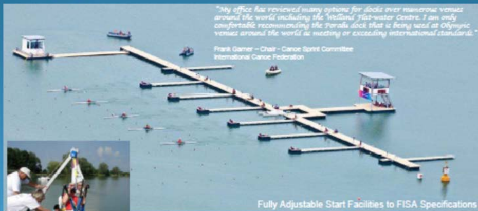
Fully Adjustable Start Facilities to FISA Specifications
